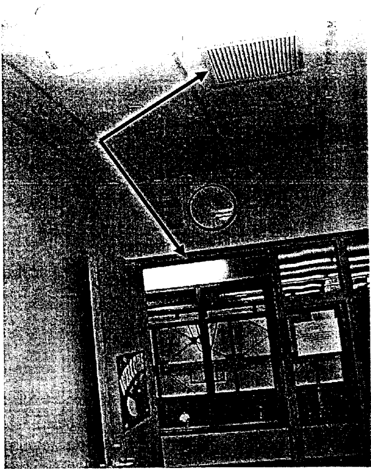
Return Vent, Note Proximity to Open Classroom/Hallway Door
