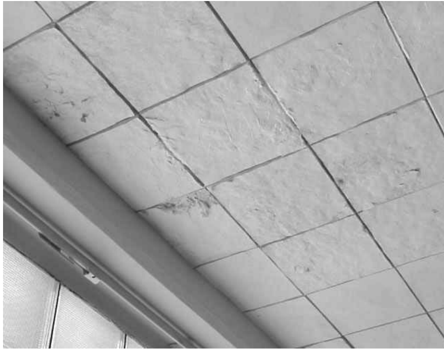
Water Damaged Ceiling Tiles around Window Frames
