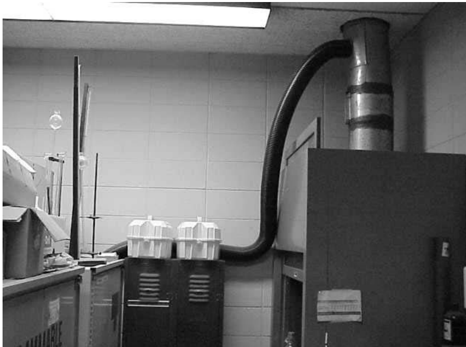
Plastic Flexible Hose Connecting Flammables Storage Cabinet to Exhaust Vent Ductwork of the Chemical Hood
