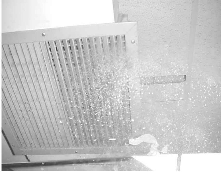
Accumulated Sawdust Knocked from Return Vent by BEHA Inspector in the Wood Shop
