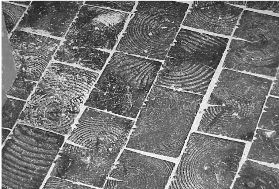
Accumulated Saw Dust in Seams of Floor Tiles in the Wood Shop
