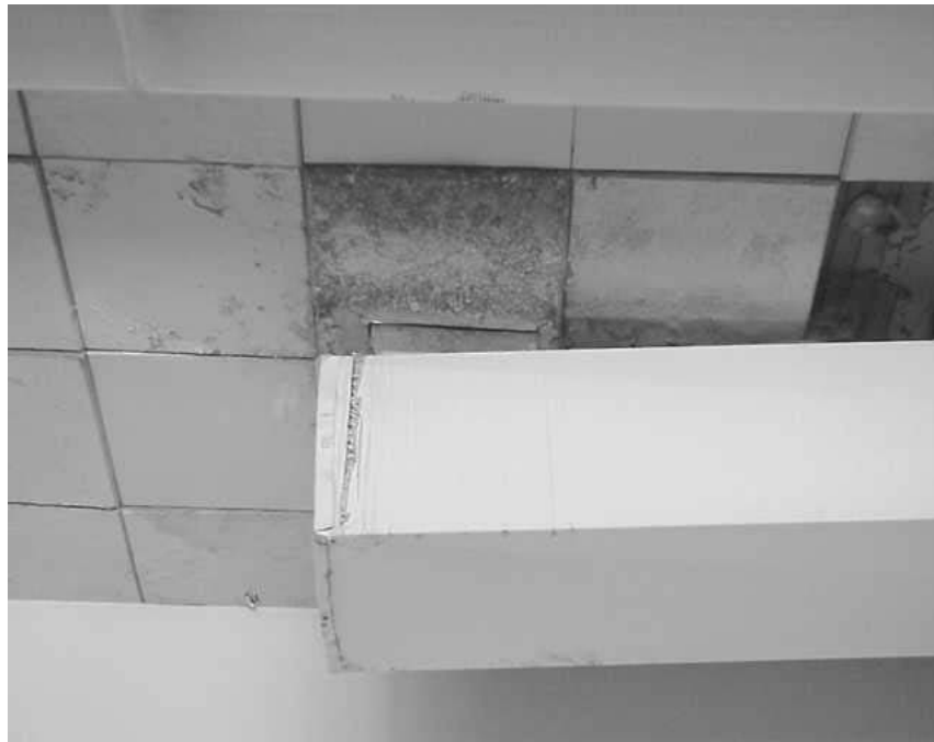
Water Damaged Ceiling Tiles around Ductwork
