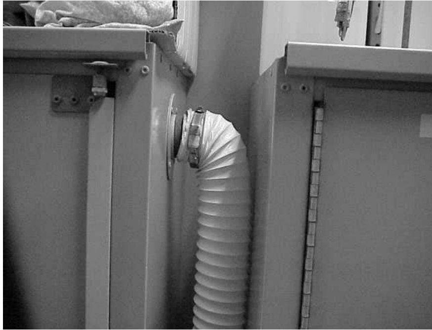
Plastic Flexible Hose Connecting Flameproof Cabinet
