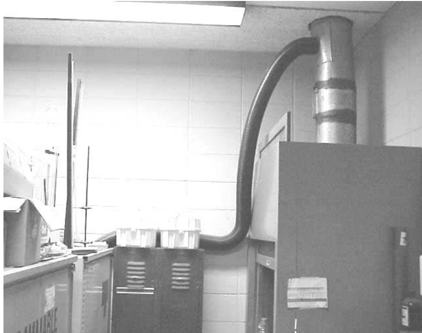
Plastic Flexible Hose Connecting Flameproof Cabinet To Chemical Hood Duct
