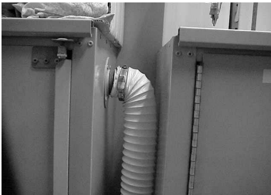
Plastic Flexible Hose Attached to Flammables Storage Cabinet Containing Volatile Organic Compounds
